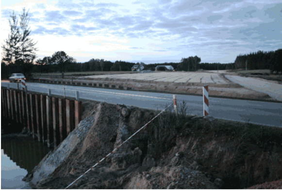
Construction work on the Augustow Bypass
